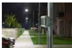
Lighting control of a residential complex and parking
